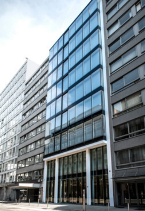
IGC Group's head office, a fully owned 9-floor office building in the heart of the Antwerp diamond district.
